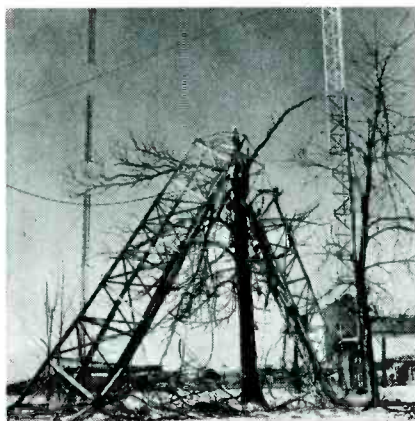
Fig. 1. Top section fell from front tower.
